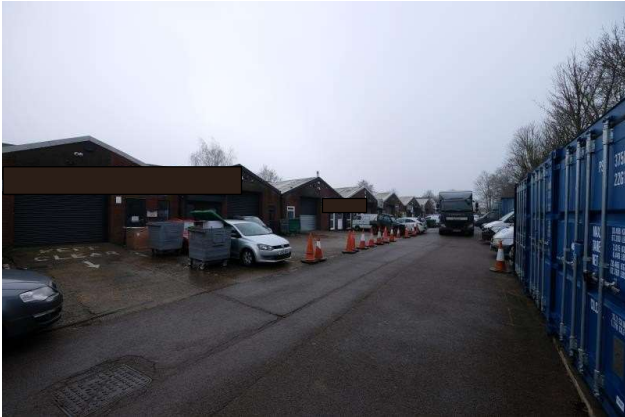
Various lock-up units at rear of but adjoining Insured's premises
