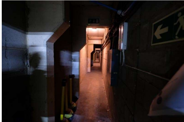
Shared fire exit corridor
