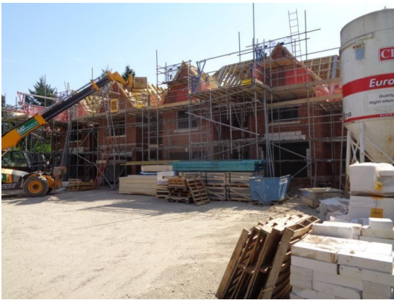
F Lane - front elevation of buildings under construction
