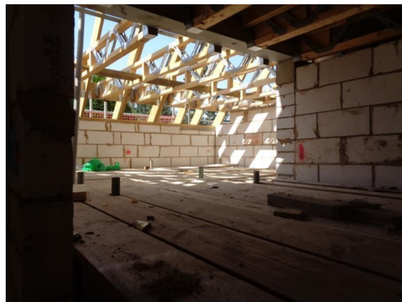
F Lane - typical interior, roof level, at this stage of construction
