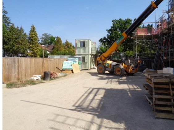
F Lane - working area to front of buildings under construction
