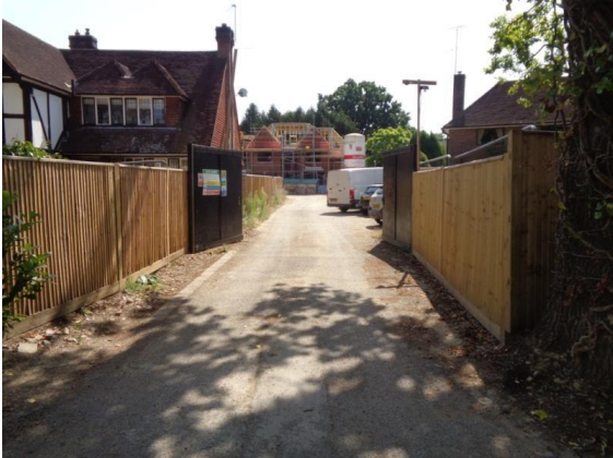
F Lane - access to site
