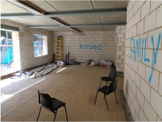
F Lane - typical interior, ground floor, at this stage of construction
